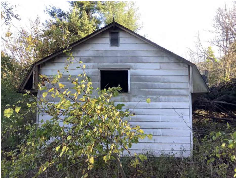
Figure 80. Photograph of 248 Stickles Road, Building 7, facing south.
