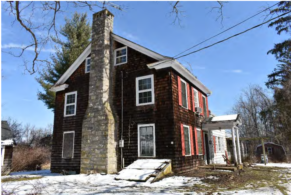
Figure 69. Photograph of 248 Stickles Pond Road, Building #5 facing northeast
