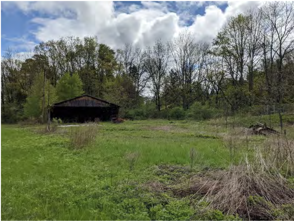
Figure 26. Wooden shed, facing east.
