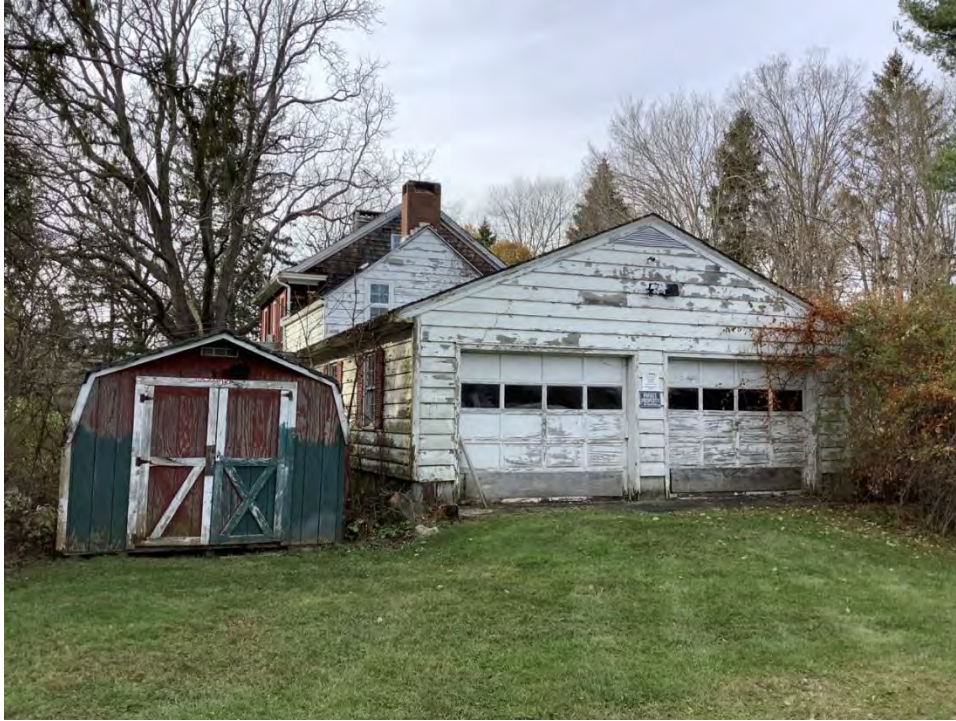
Figure 66. Photograph of 248 Stickles Pond Road, Building #5, facing west.
