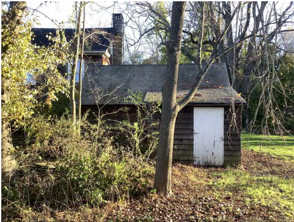
Figure 78. Photograph of 248 Stickles Road, Building 6, facing south.
