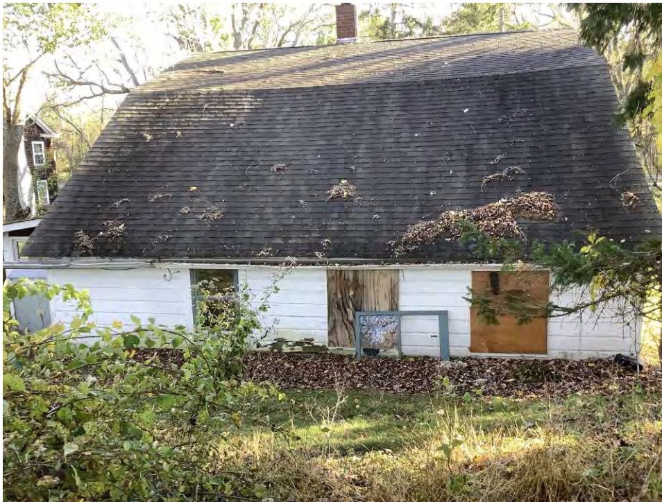
Figure 61. Photograph of 248 Stickles Road, Building #4, facing south.
