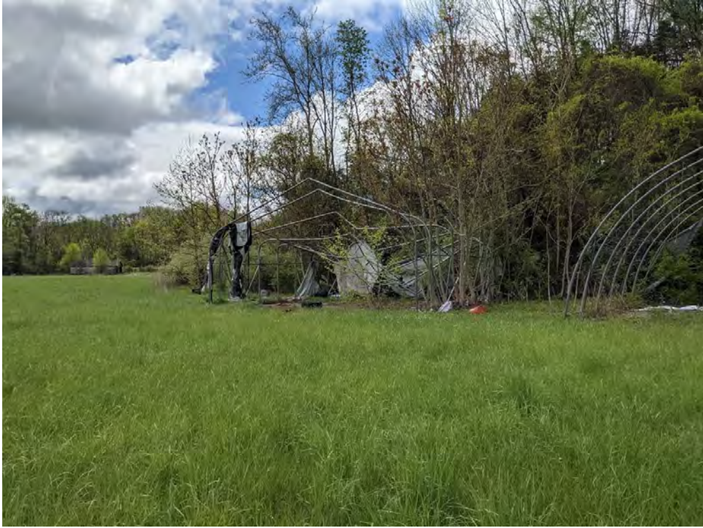
Figure 25. Two abandoned tent structures on west side of X-shaped area, facing south.
