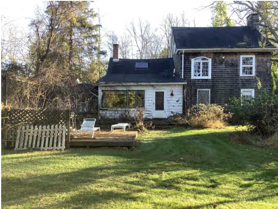
Figure 67. Photograph of 248 Stickles Pond Road, Building #5, facing south.
