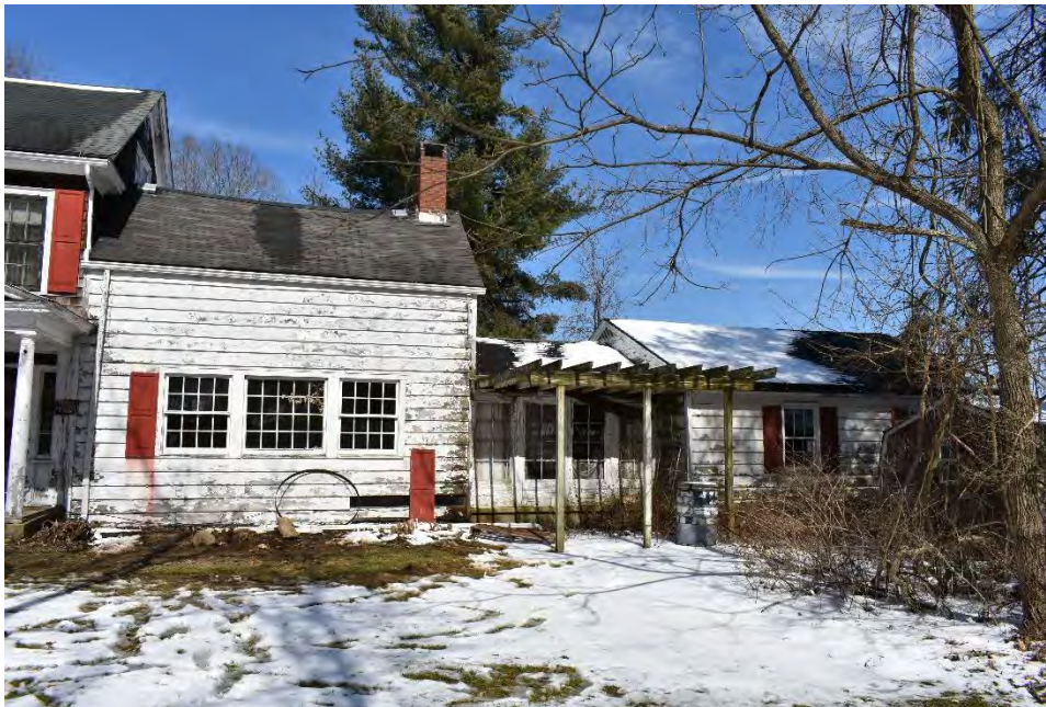
Figure 65. Photograph of 248 Stickles Pond Road, Building #5, facing north.
