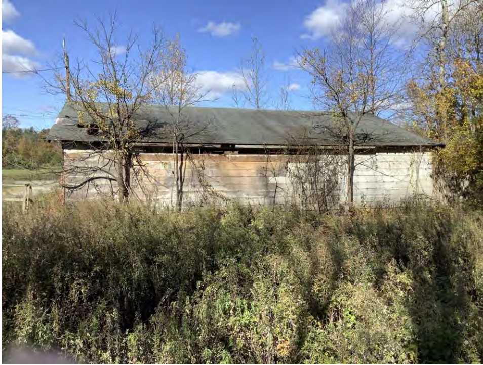
Figure 54. Photograph of 248 Stickles Pond Road, Building #2, facing north.
