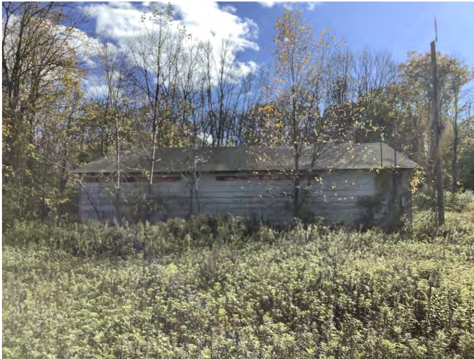
Figure 51. Photograph of 248 Stickles Pond Road, Building #2, facing south.
