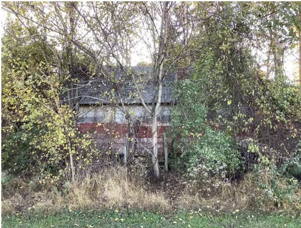
Figure 82. Photograph of 248 Stickles Road, Building 7, facing west.
