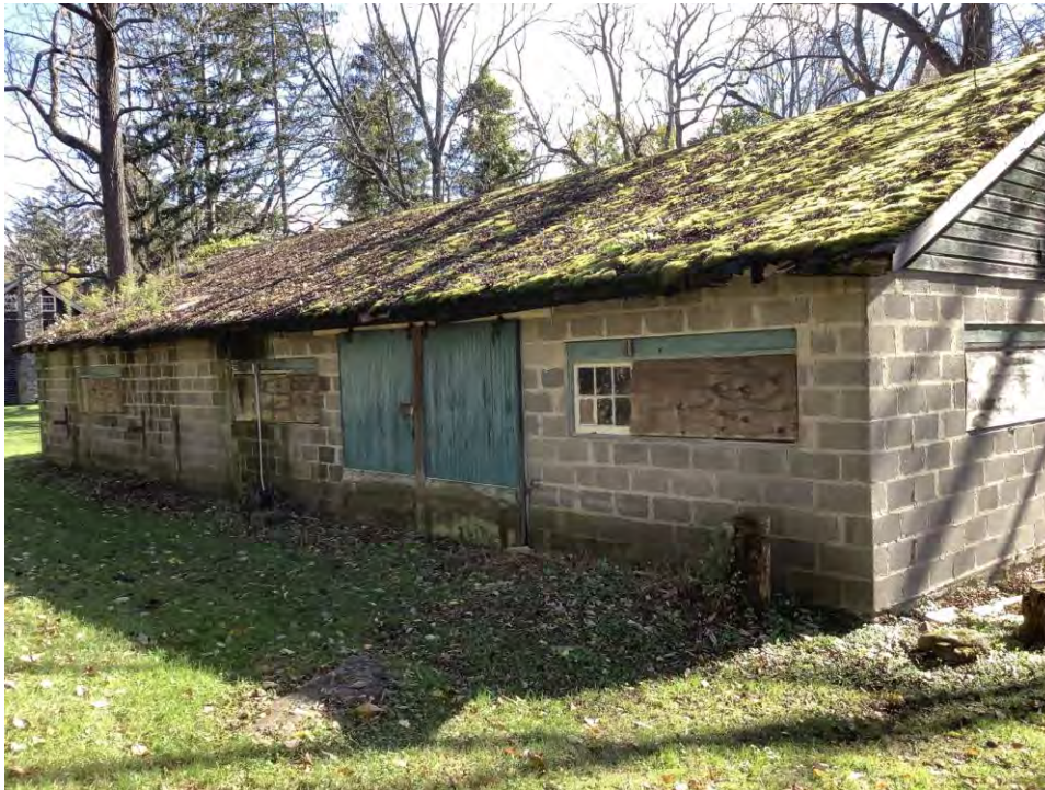
Figure 49. Photograph of 248 Stickles Road, Building #1, facing south.
