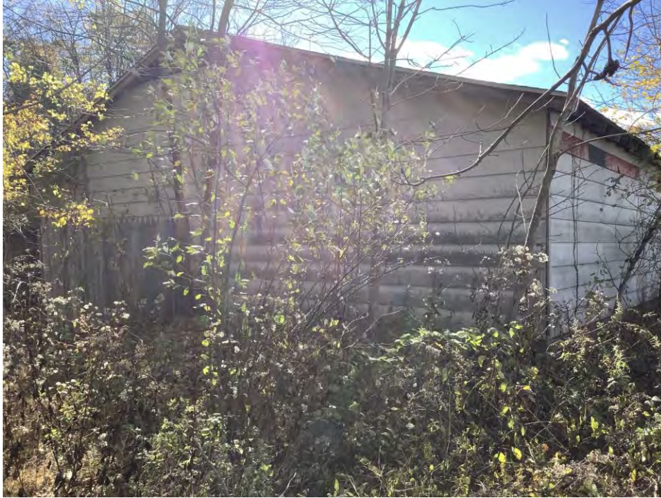
Figure 52. Photograph of 248 Stickles Pond Road, Building #2, facing southwest.
