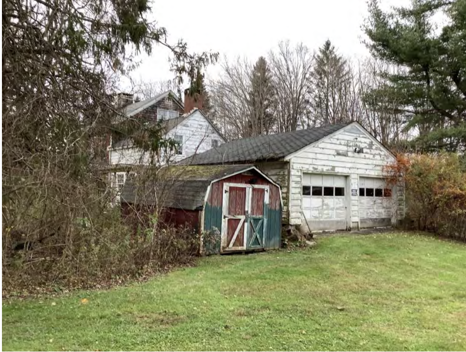
Figure 83. Photograph of Building #8 - Shed, facing west.
