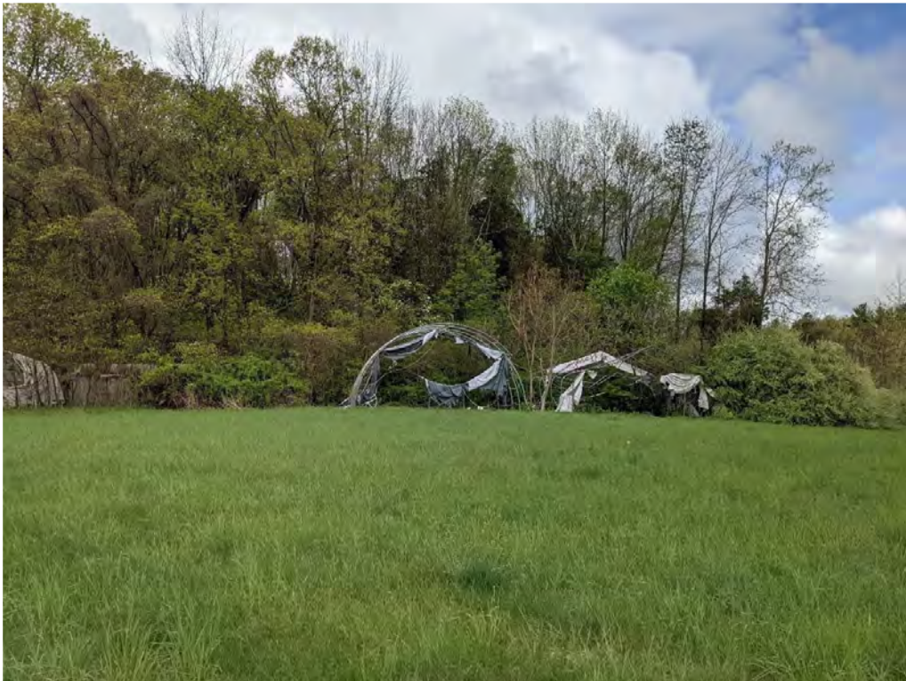
Figure 24. Three abandoned tent structures on west side of X-shaped area, facing west.
