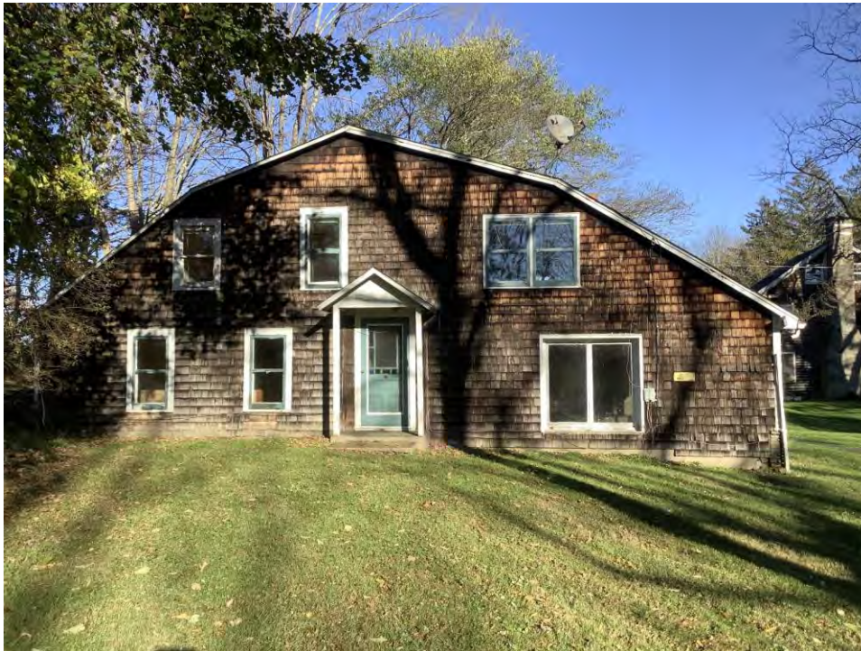
Figure 59. Photograph of 248 Stickles Road, Building #4, facing east.
