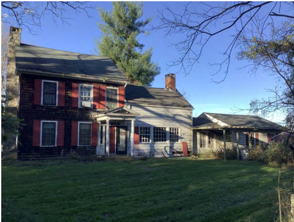
Figure 63. Photograph of 248 Stickles Pond Road, Building #5, facing northeast.
