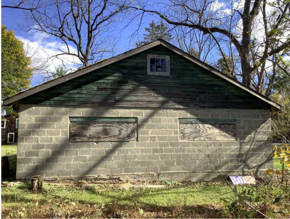
Figure 48. Photograph of 248 Stickles Road, Building #1, facing east
