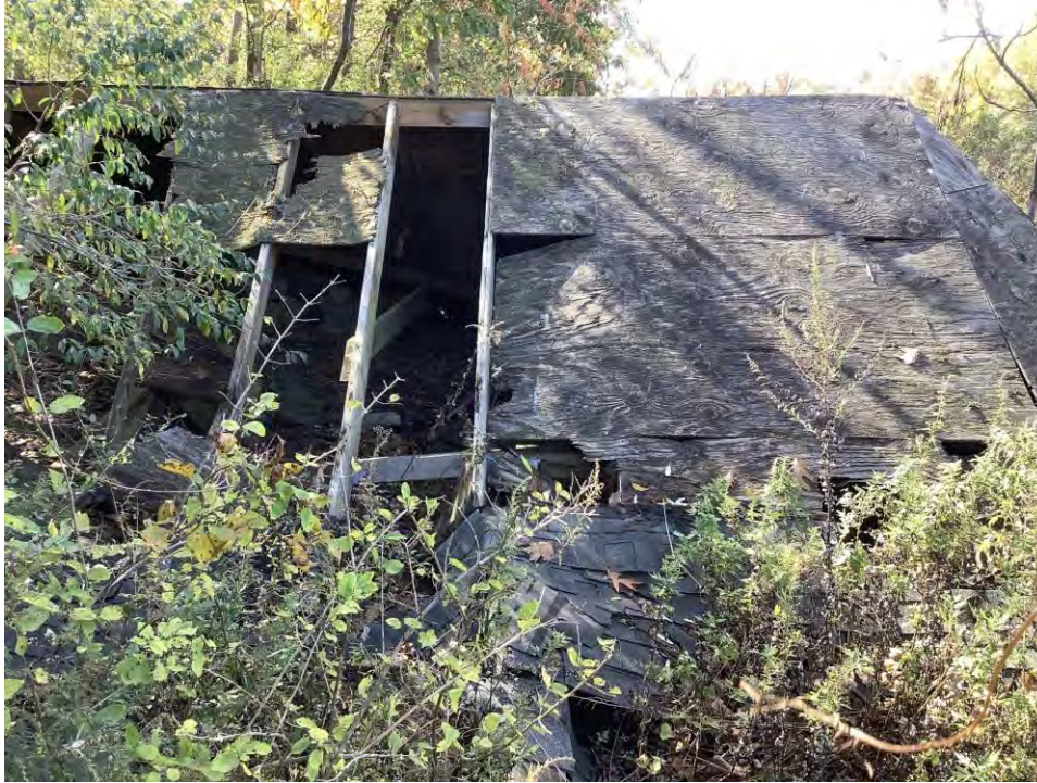
Figure 56. Photograph of 248 Stickles Pond Road, Building #3, - 1, facing west.
