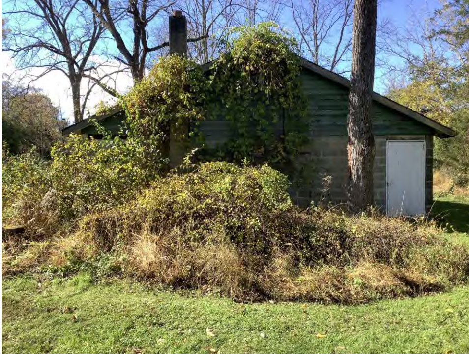
Figure 50. Photograph of 248 Stickles Road, Building #1, facing west.
