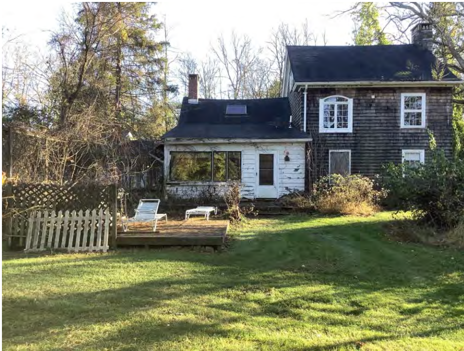
Figure 71. Photograph of 248 Stickles Pond Road, Building #5, facing south.
