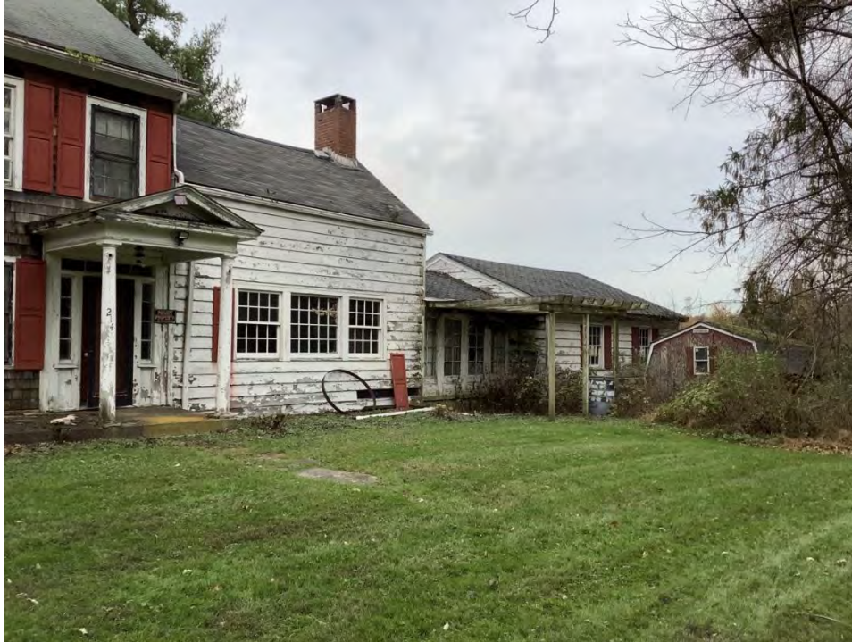
Figure 64. Photograph of 248 Stickles Pond Road, Building #5, facing northeast.
