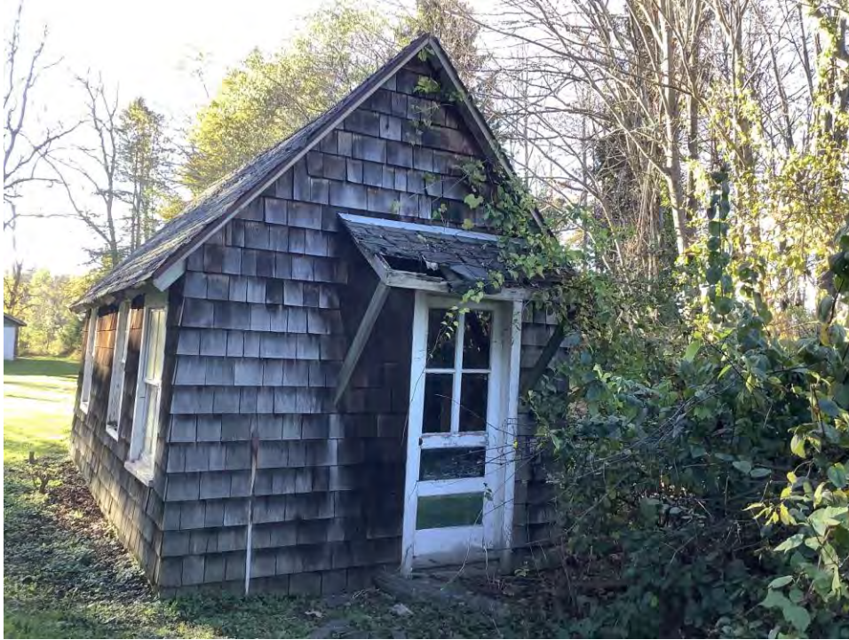
Figure 75. Photograph of 248 Stickles Road, Building 6, facing east.
