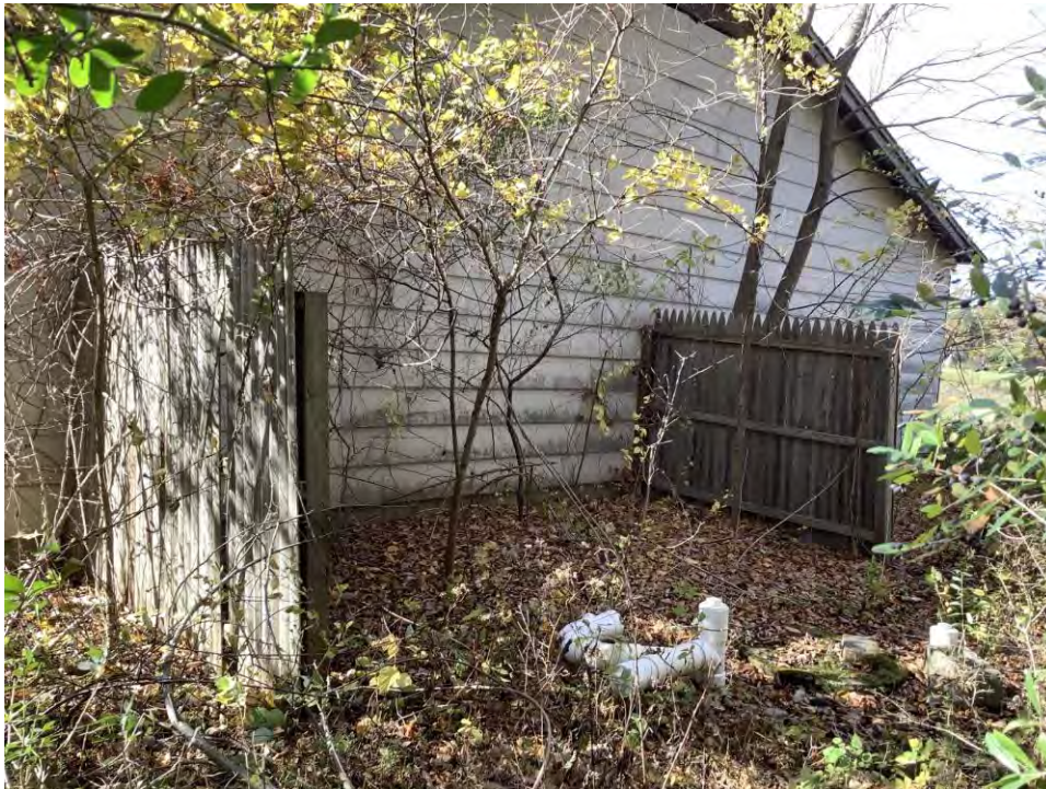
Figure 53. Photograph of 248 Stickles Pond Road, Building #2, facing northwest
