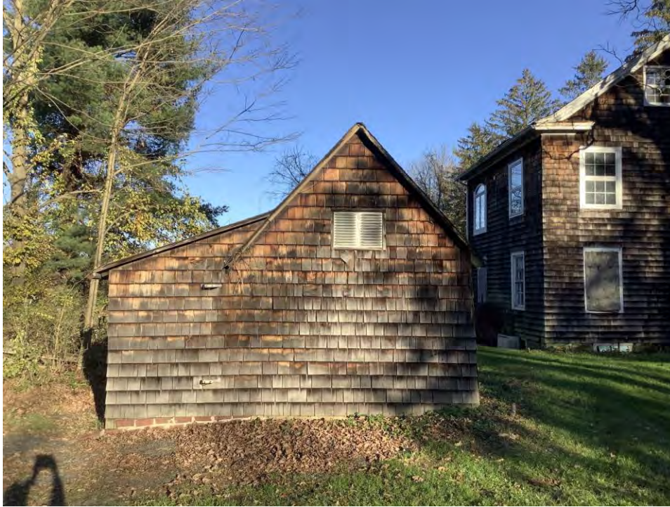
Figure 77. Photograph of 248 Stickles Road, Building 6, facing east.
