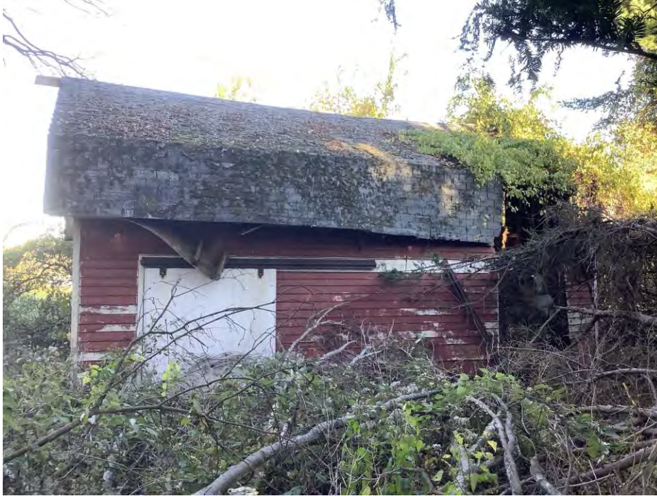
Figure 79. Photograph of 248 Stickles Road, Building 7, facing east.
