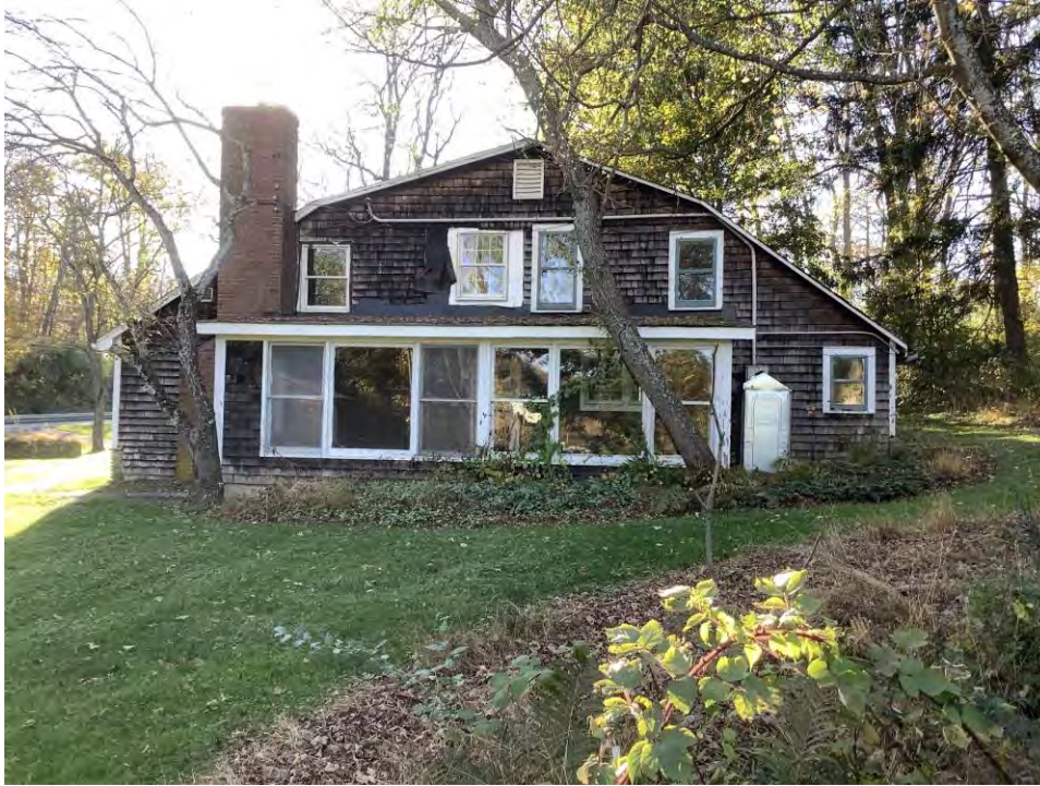
Figure 62. Photograph of 248 Stickles Road, Building #4, facing west.
